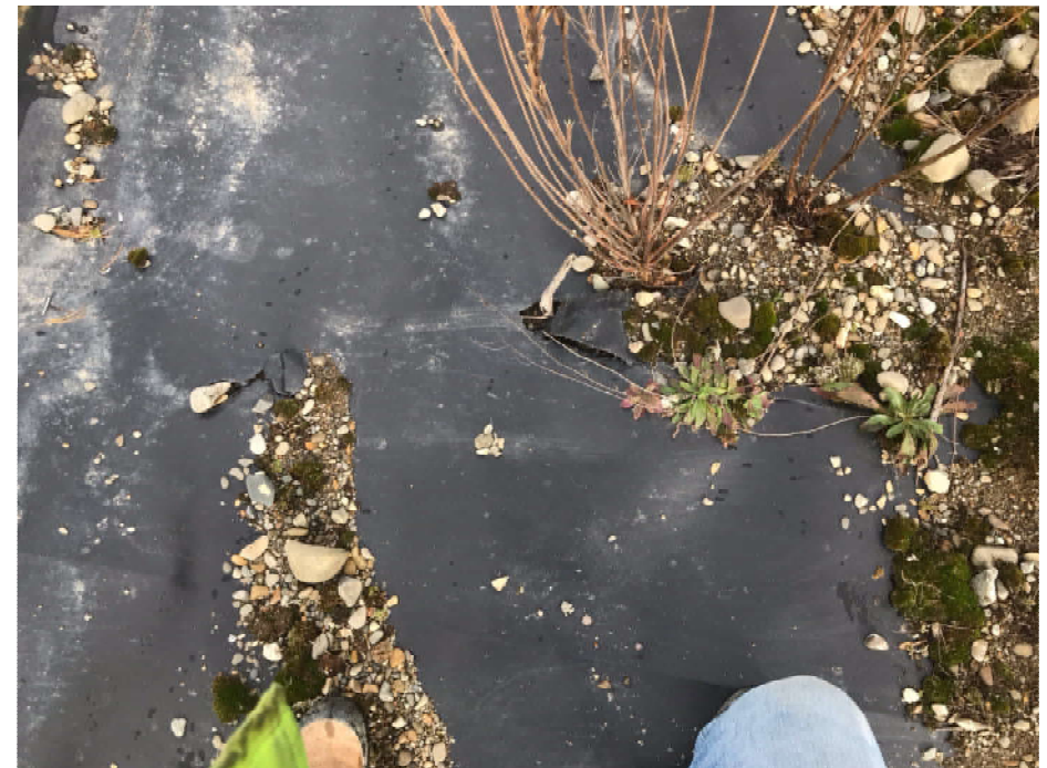
Hole in Lagoon Liner
