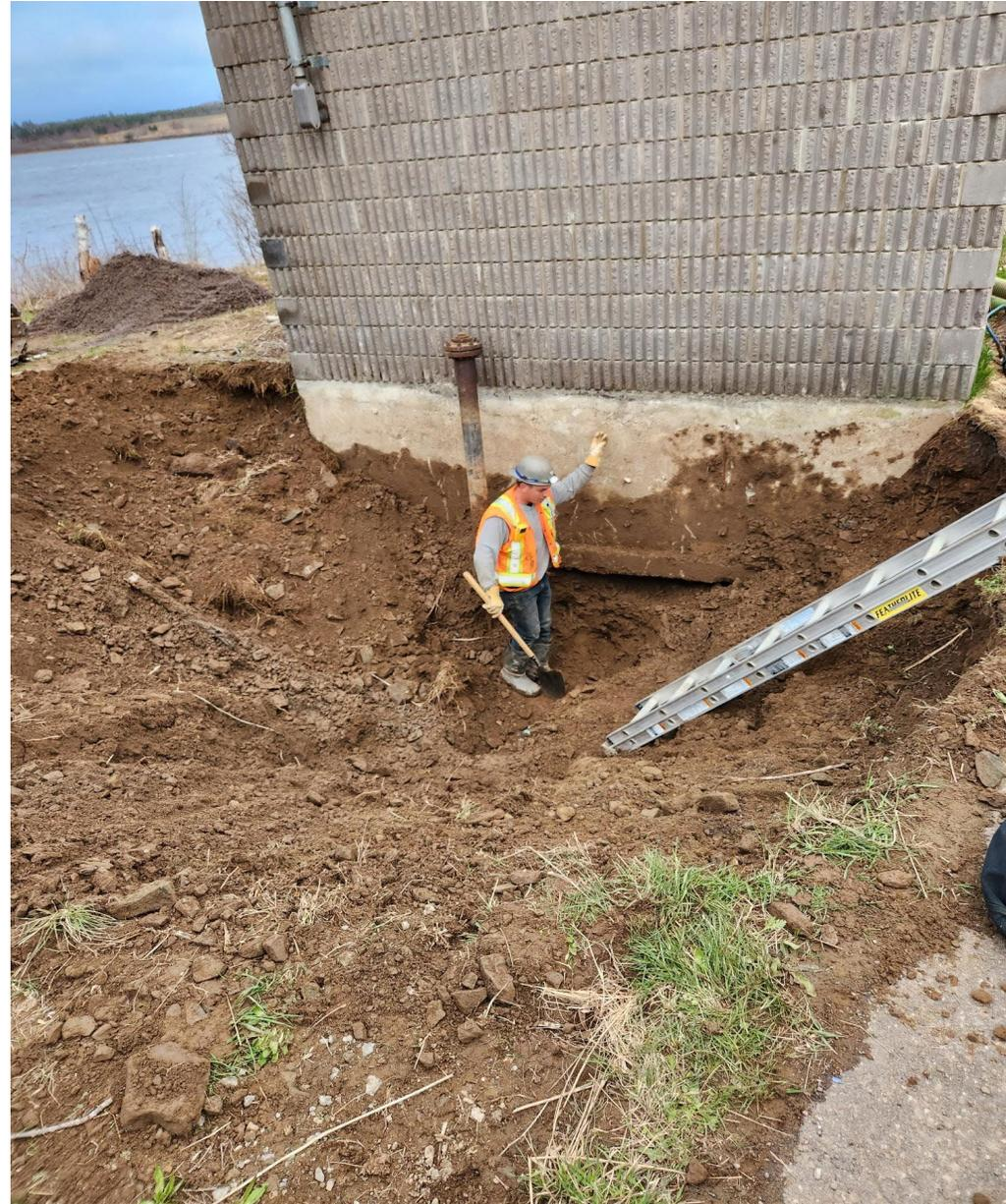
In stable rock and **engineer approved** soil conditions, a straight walled trench may be permissible. This is to be the exception not the rule and a ladder must be used. Wire netting can also be used to protect operators from falling rock, debris.
